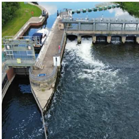
St Ives Lock and Sluice showing how the stream from the sluice in strong flows, can push boats against the bulge in the entrance wall.
