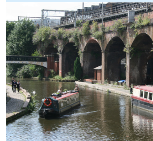
The Bridgewater canal at Castlefield Photo: Peter Fellows
