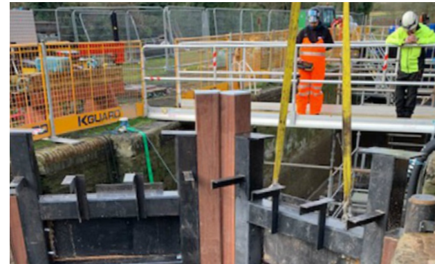
Composite lock gate being trialled at Picketsfield Lock Photo: CRT
