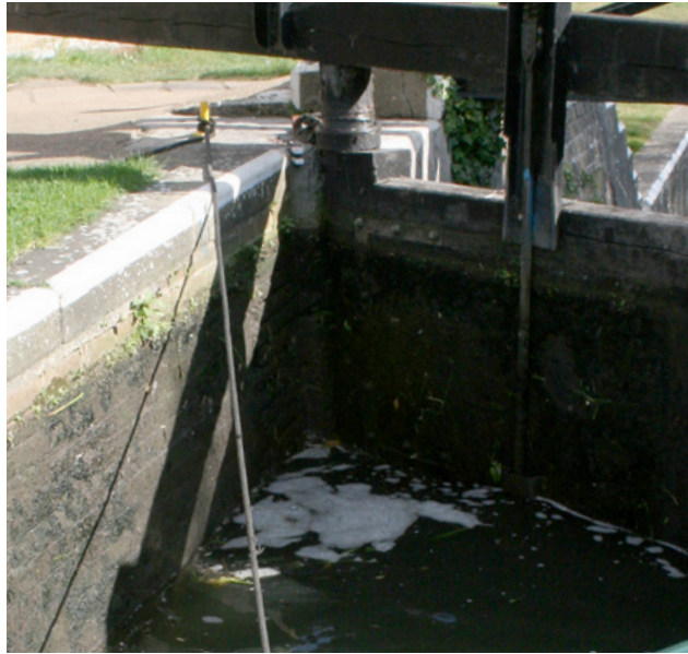
Using the yellow spike for a stern rope going down
