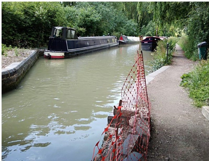
Bridge deconstruction to allow a widebeam to pass. Photo: Mark Tizard
