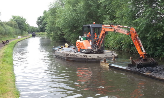
Dredging on the Staffs & Worcs Canal
