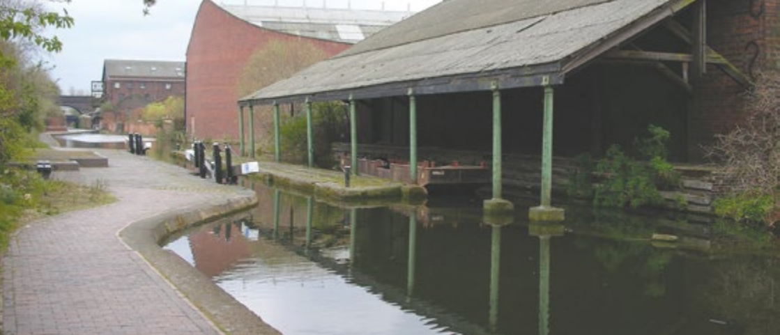
Warwick Bar stop lock and banana warehouse
