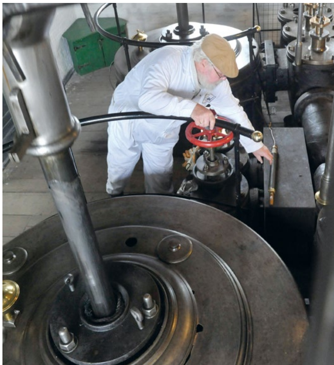
Dick Poole operating the Crofton beam engine
