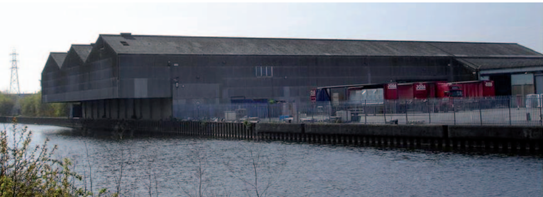
CRT Leeds Inland Terminal at Knostrop
