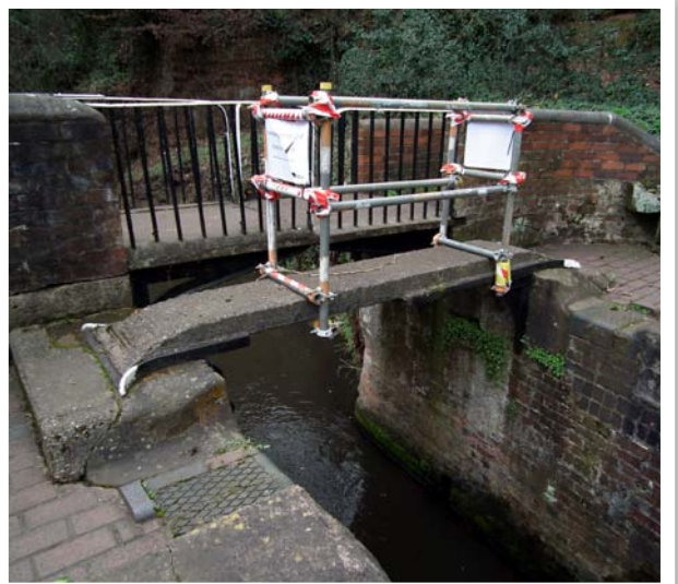
Concrete bridge at Caldwell Lock Photo: Fiona Slee
