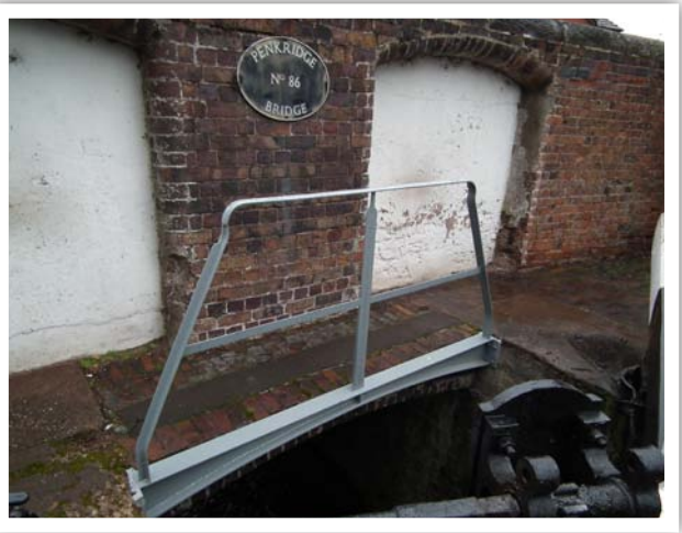
New rails on tail bridge at Penkridge Lock Photo: Fiona Slee
