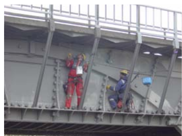
Engineers examine Benjamin Bevan's aqueduct crossing the Great Ouse at Wolverton Photos Geoff Wood
