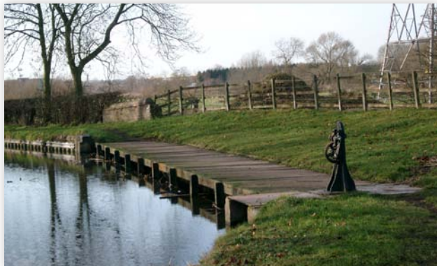
The site of the entrance to the Stafford Branch Canal from the Staffs & Worcs Canal showing the left hand remains of the roving bridge over the junction.
