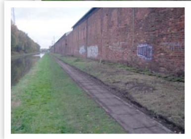
Before and after: towpath widening on the Tame Valley Canal
