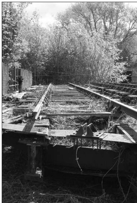
Heritage or junk? The remains of the swingbridge in the Sheepwash channel on the approach to the Oxford Canal from the Thames
