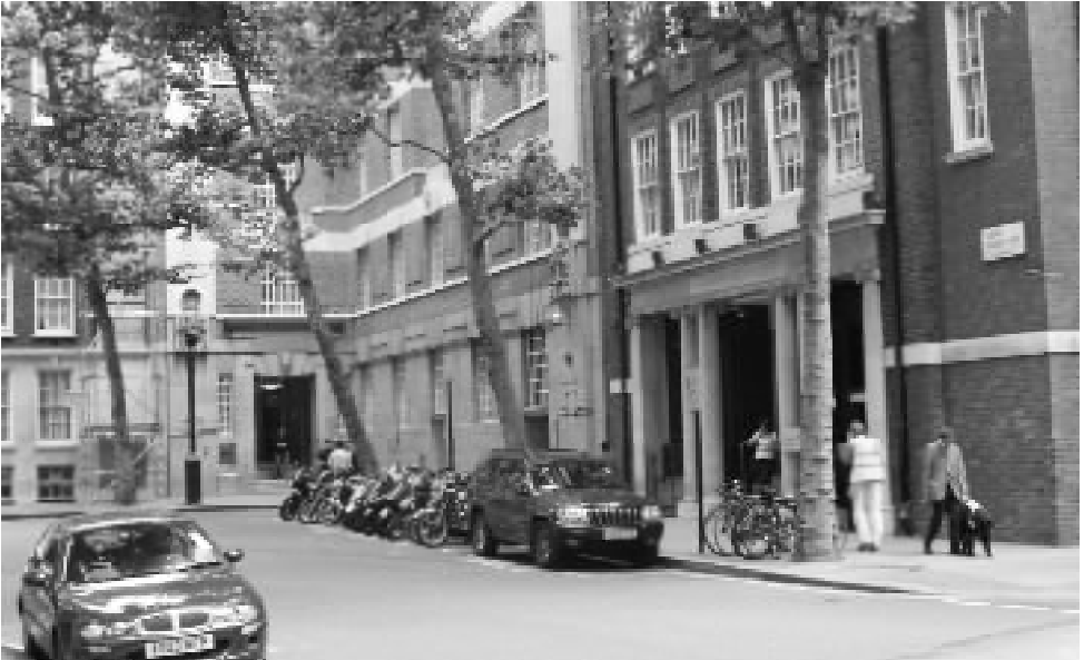
The tree lined corner of Smith Square where waterway decisions are made, DEFRA’s Nobel House. Transport House is to the right of it.
