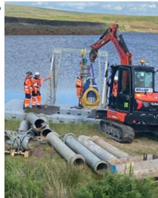
Photo 5: Submersible pump lifted to moonpool
