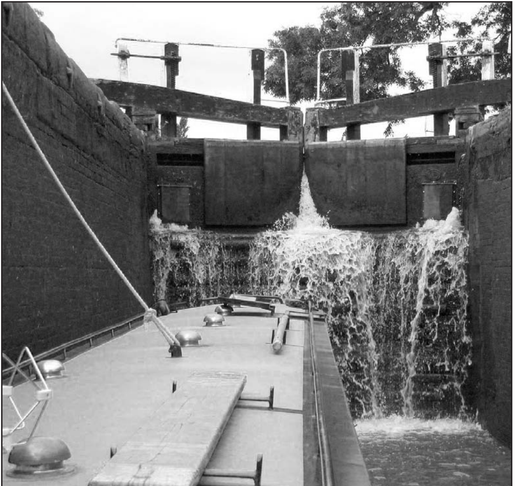
Top gate waterfall at Stenson Lock, Trent and Mersay Canal. Photo: Sir Ron Nella
